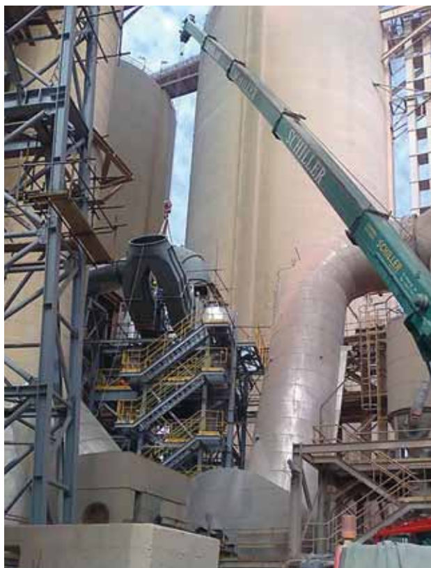
Figure 6: installing HGD supports in between existing structures
