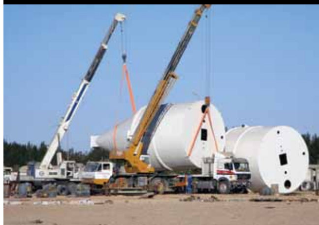
Figure 5: delivering preassembled 200m³ raw coal silos
