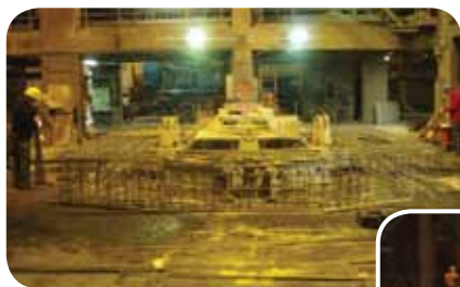
Figure 4 (above): the new foundation placed onto the existing floor rather than embedded in the ground
