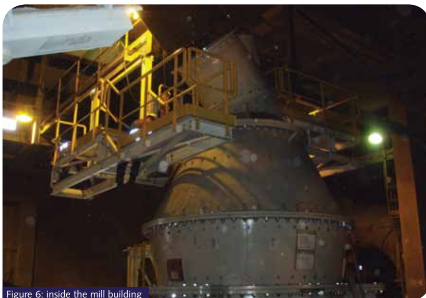
Figure 6: inside the mill building
