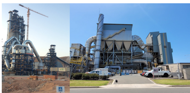
Figure 1. Plants with MVR 6000 R-6 mills: Bag filter system (right), cyclone dust separation (left).
