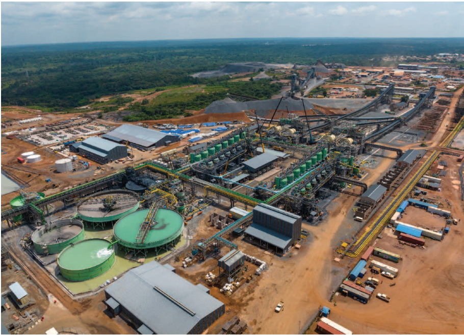
CITIC HIC supplied four sets of \Phi 6.1 \times 9.75 m ball mills to bring processing capacity at the Kamoakakula mine up to 7.6 Mt/y as part of the development of Phases 1 & 2 (photo: Ivanhoe Mines)
