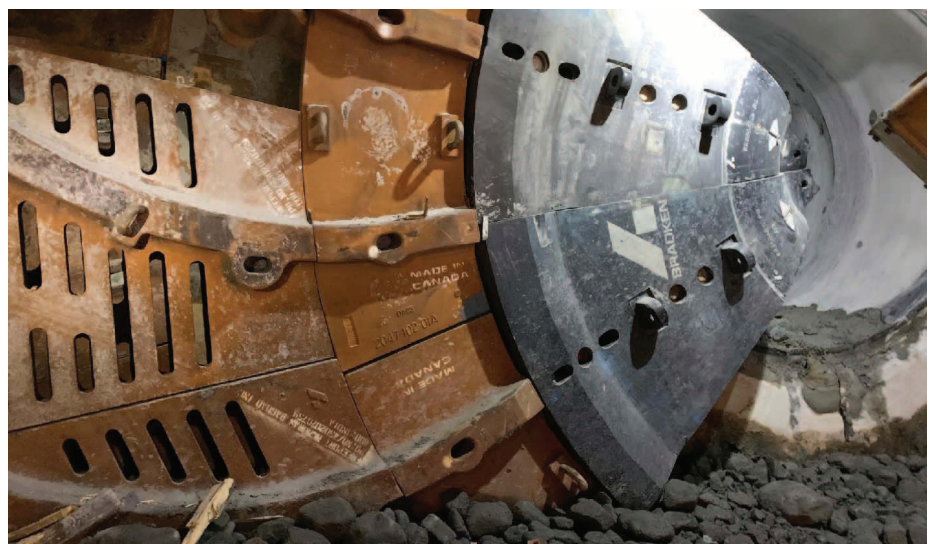
A half-row double-wide Bradken Vortex discharge system was behind a 9.5% throughput increase and a 2.5% reduction in overall circuit energy consumption at the Bagdad mine
