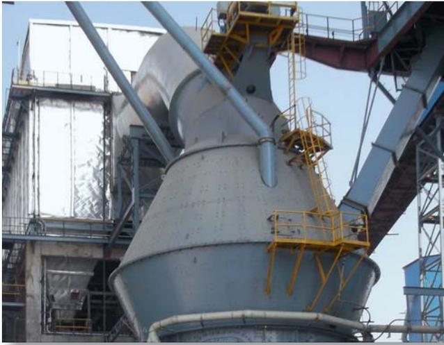
Figure 4: Feeding points for fly ash at the upper classifier housing
